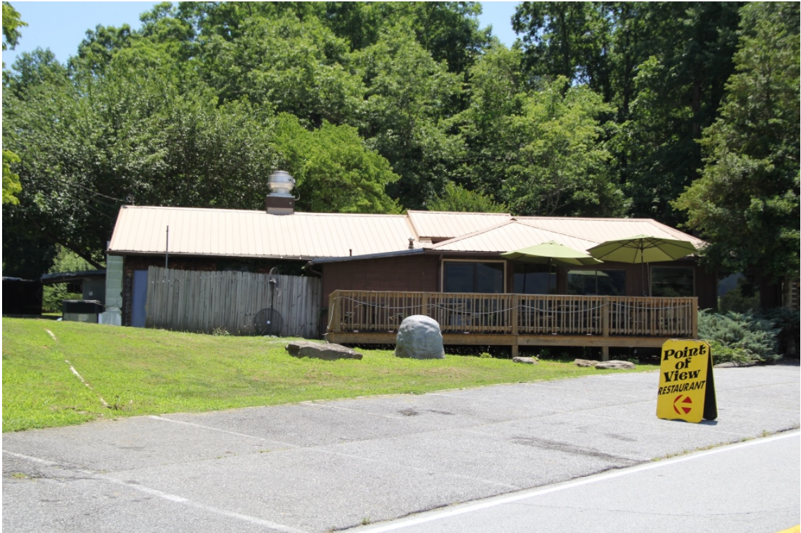
The Log Shop, 454 Memorial Highway, side elevation, view to southeast
