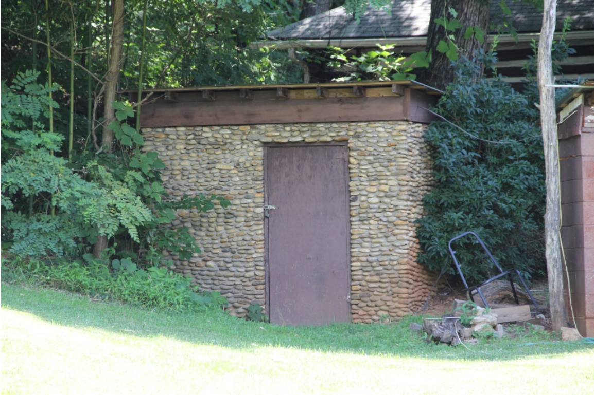
Storage building, ca. 1930s, view to southwest
