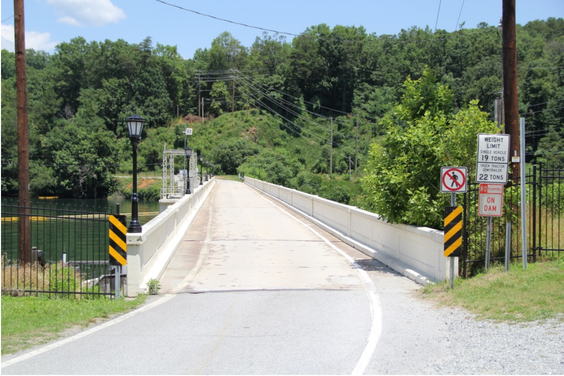
Bridge No. 628 over Lake Lure Dam, view to north
