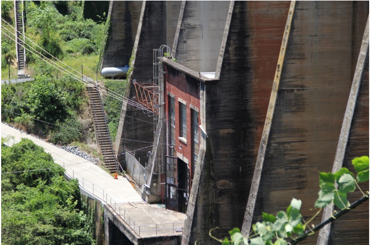
Lake Lure Hydroelectric Plant, view to southwest
