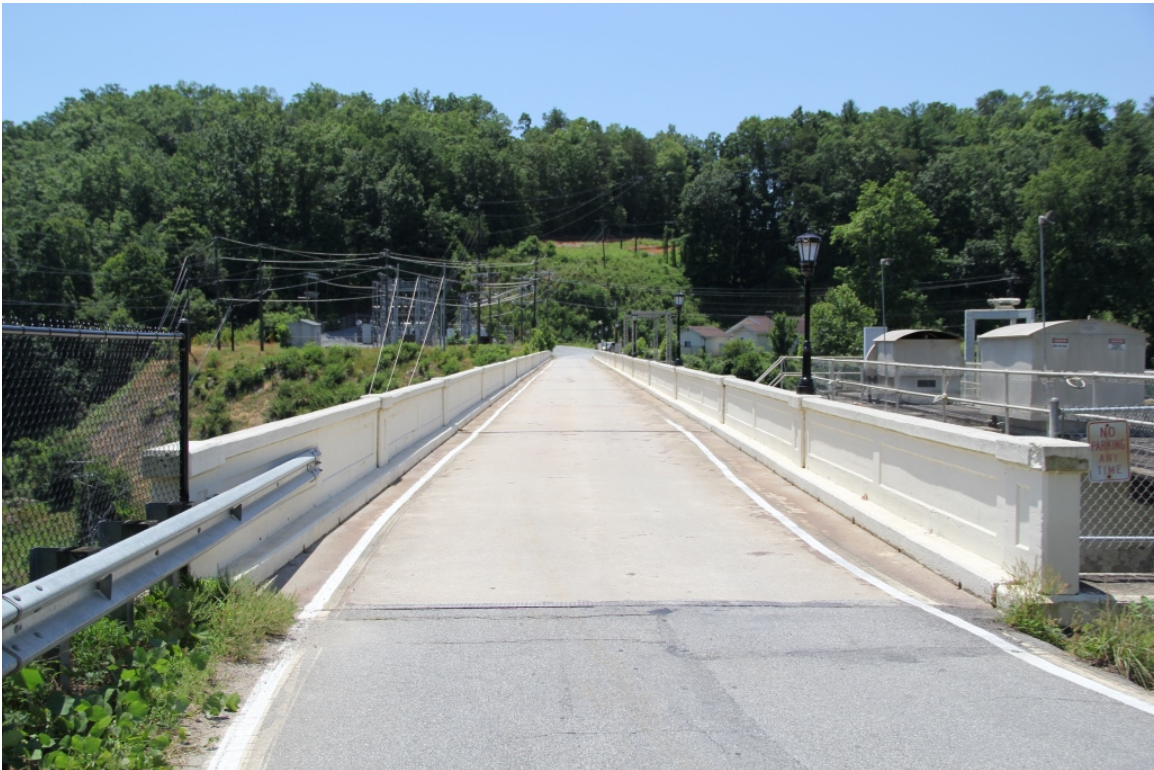
Bridge No. 628 over Lake Lure Dam, view to south
