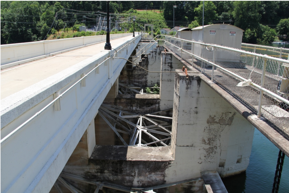
Lake Lure Dam, spillway gates, view to south
