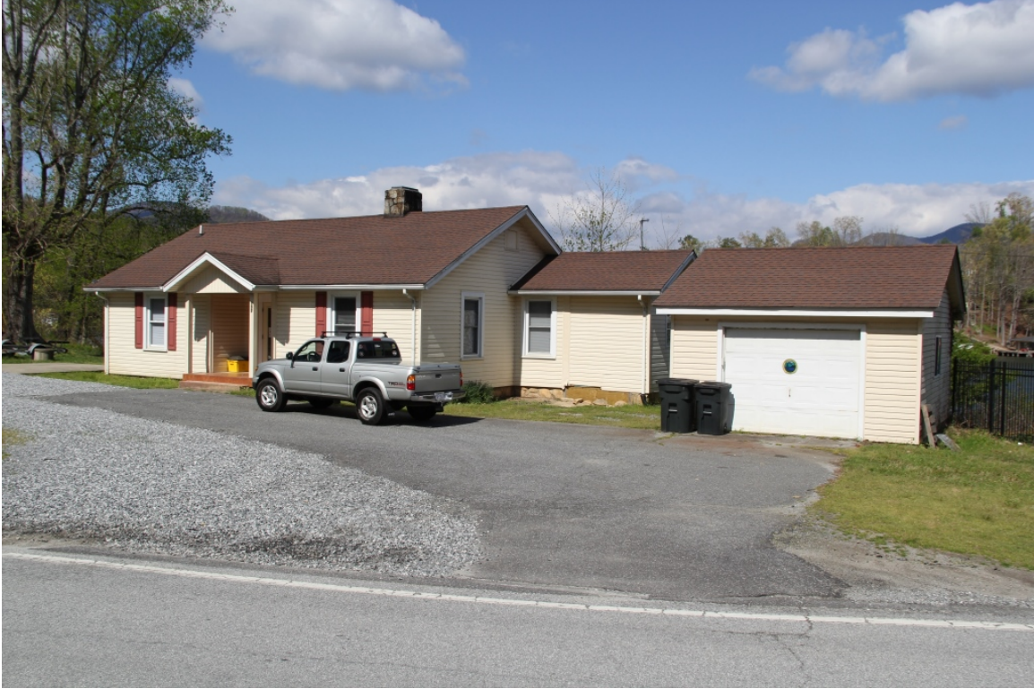
Dam Operator's House and garage, view to west (April 2016)
