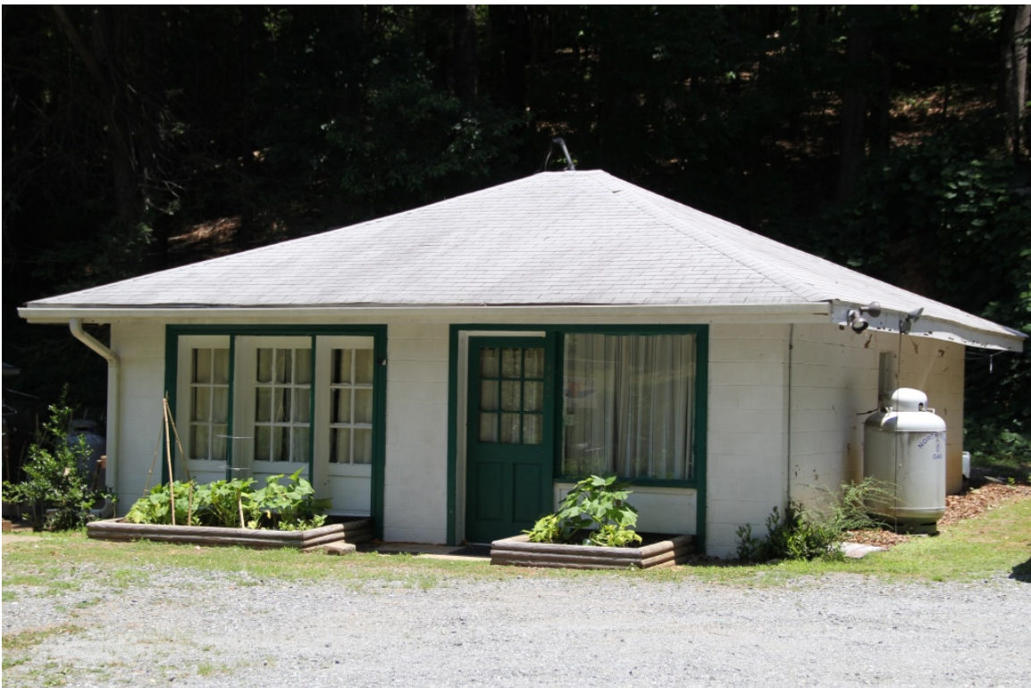
L. M. Pearson Realty Office, 442 Memorial Highway, façade, view to north
