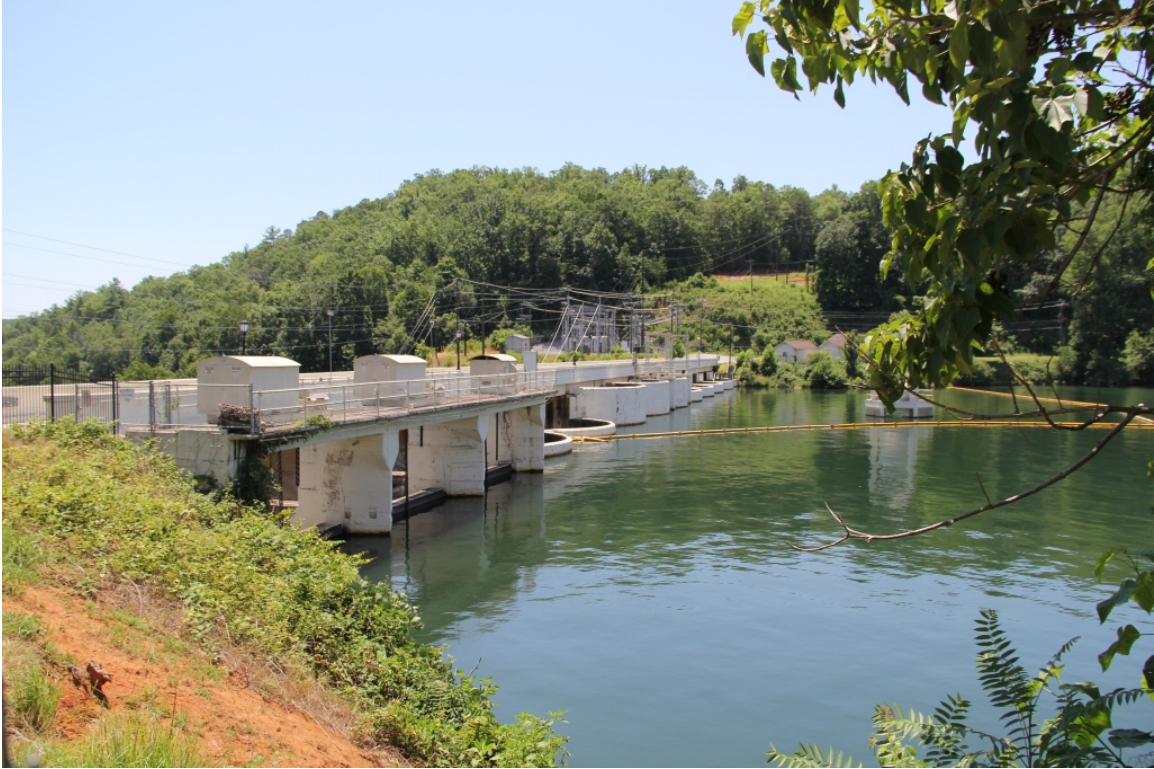
Lake Lure Dam, view to southeast
