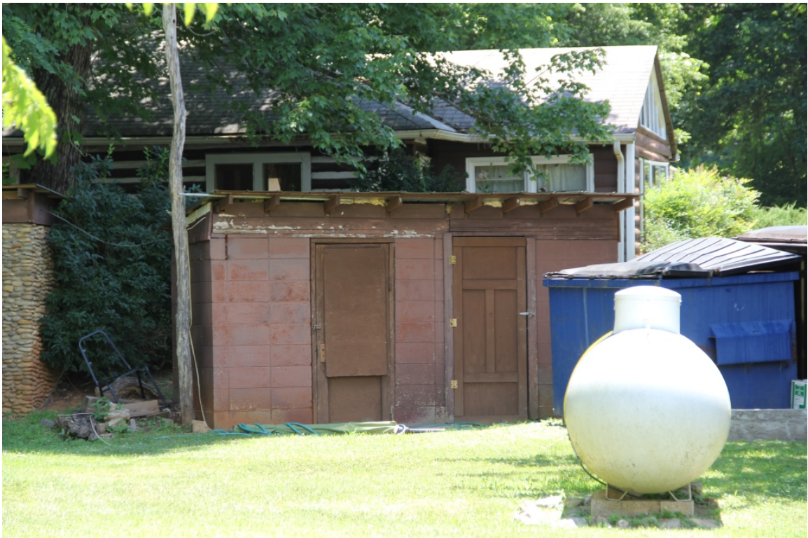
Storage building, ca. 1950s, view to southwest
