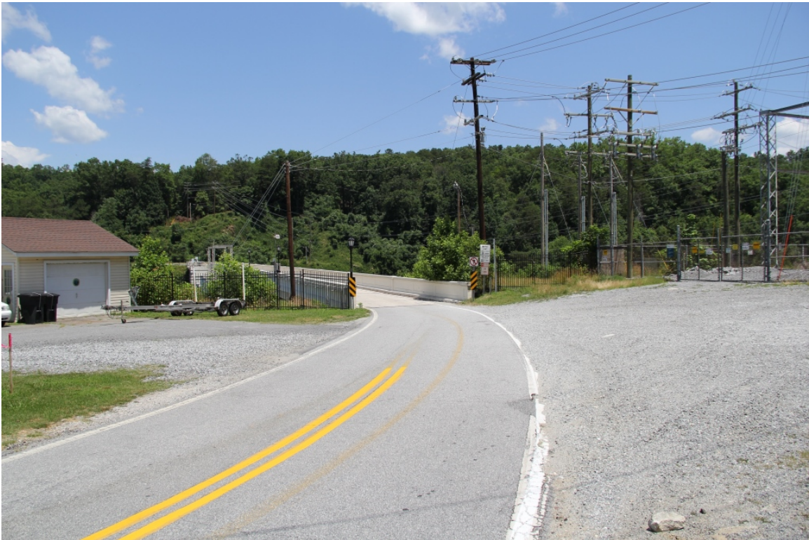
Bridge No. 628, view to northeast on Buffalo Shoals Road (SR 1306)
