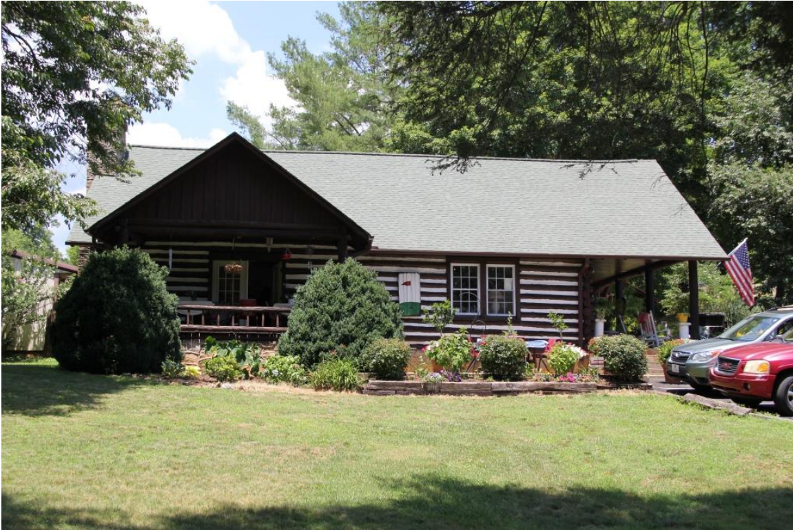
Clubhouse, Lake Lure Golf Course, 658 Memorial Highway, side elevation, view to northwest
